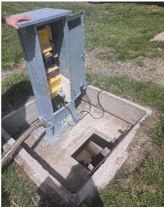
Photo 6 – existing snowmaking pit requiring drainage
